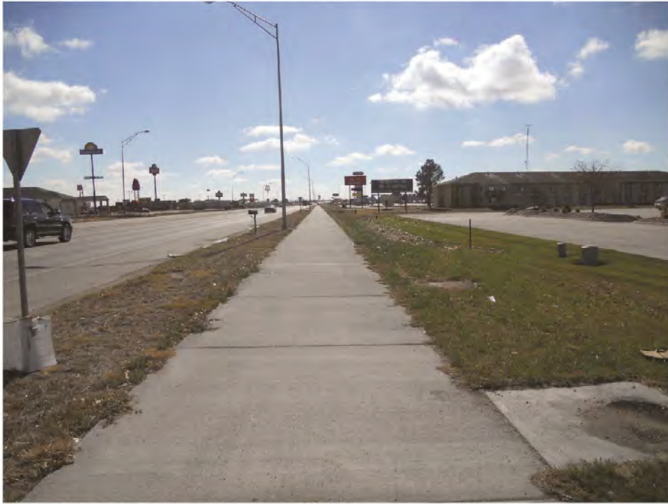
Existing Conditions along Plum Creek Parkway
